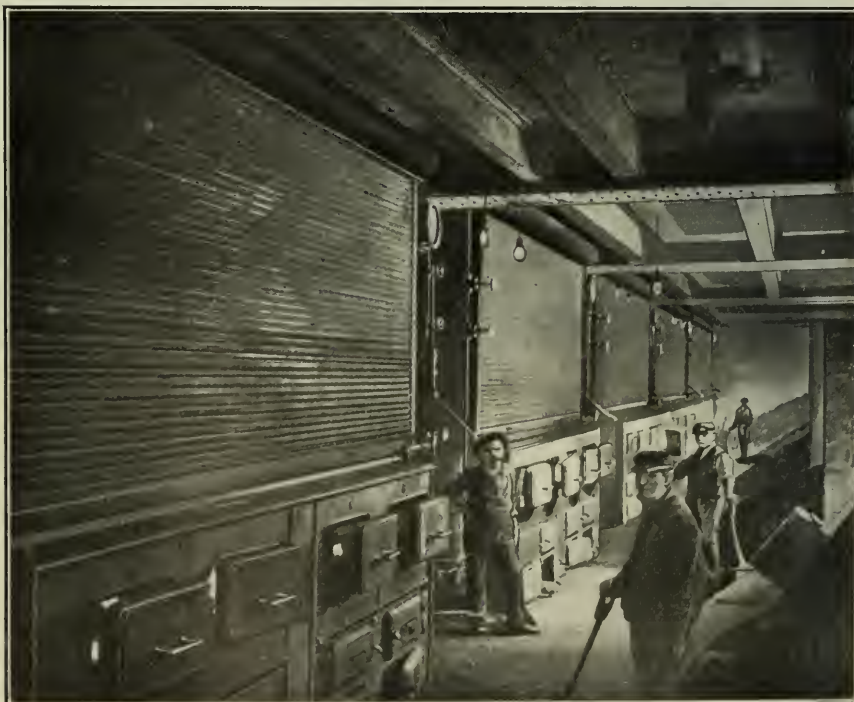
FIG. 3. VIEW IN BOILER ROOM
